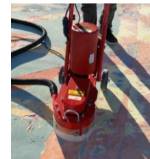
④ Decontamination through mechanical stripping (floor surfaces)
