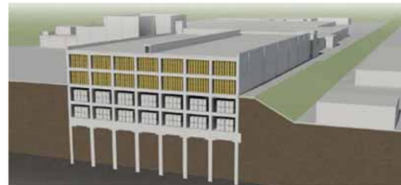
Storage floor selected in accordance with the surface dose rate (example: >30mSv/h waste stored on subfloor 2) (Current plan calls for the facility to be used to store rubble)
