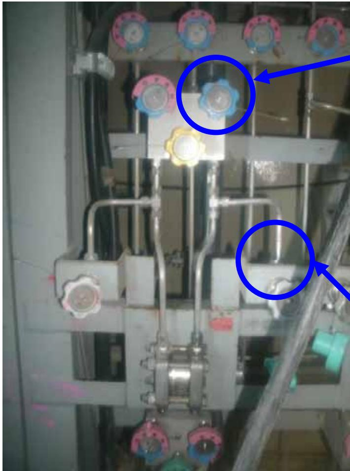
Rack for Jet Pump Measurement
