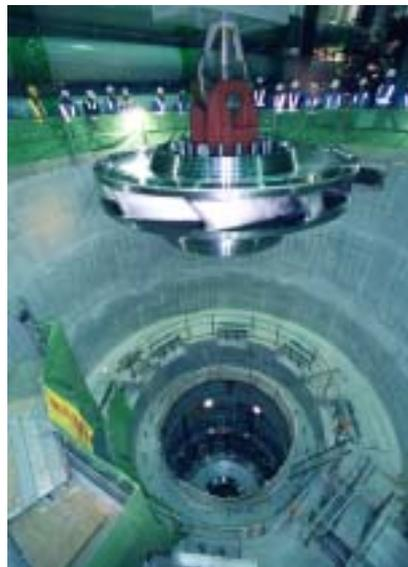
**On-site work to install the pump-turbine runner**
