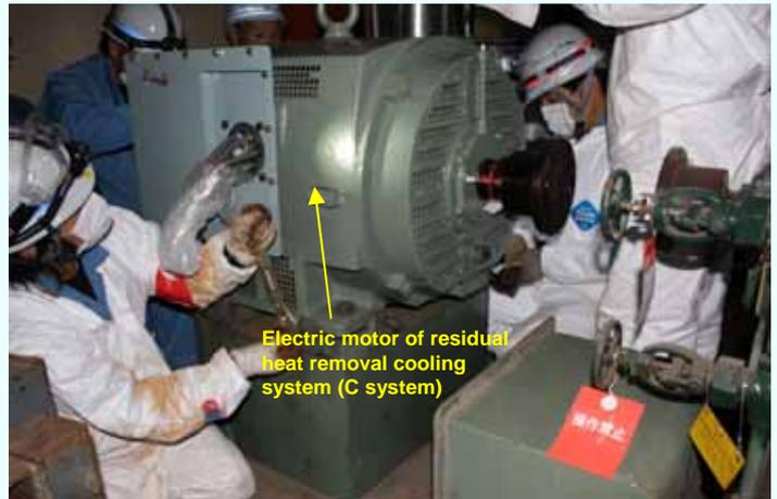
Installing the electric motor of residual heat removal cooling system (C system): Enlarged image
