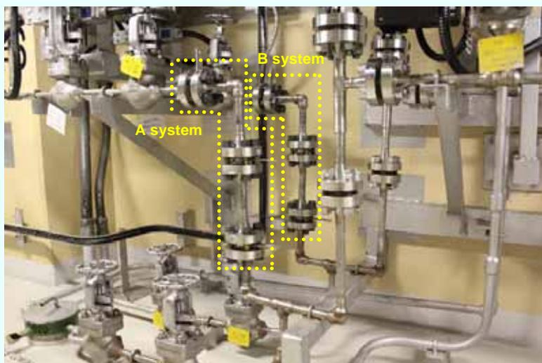
Purge line (A system, B system) after being switched to the permanent pipe [Completed on October 11, 2012] (Photo taken on October 29, 2012)
