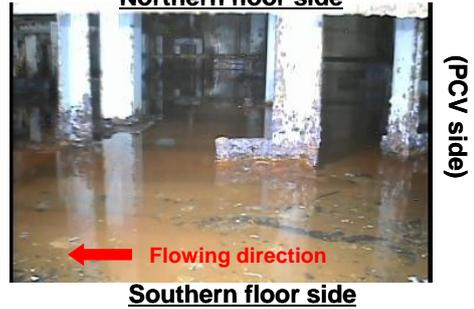
Figure 4-3 Water leaks from main steam line D in MSIV room
